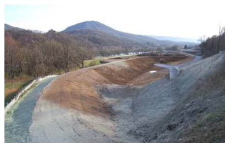
Fly Ash Site along the New River in Giles.
